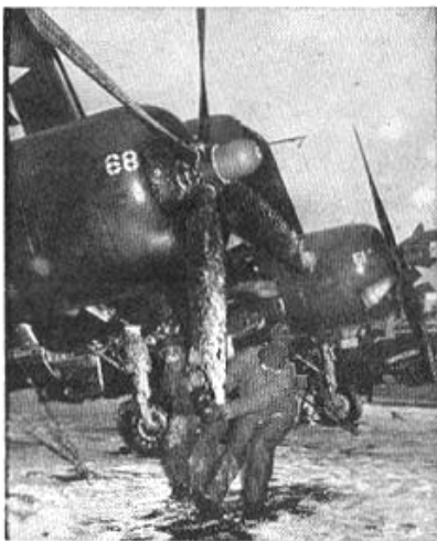
MOTORS START SLOWLY and with difficulty in planes stored on flight deck. Hangared planes did better.
